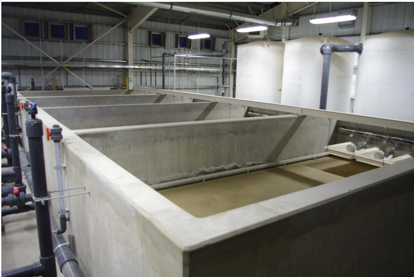
Inside Exshaw water treatment plant showing four filters and three contact tanks.
