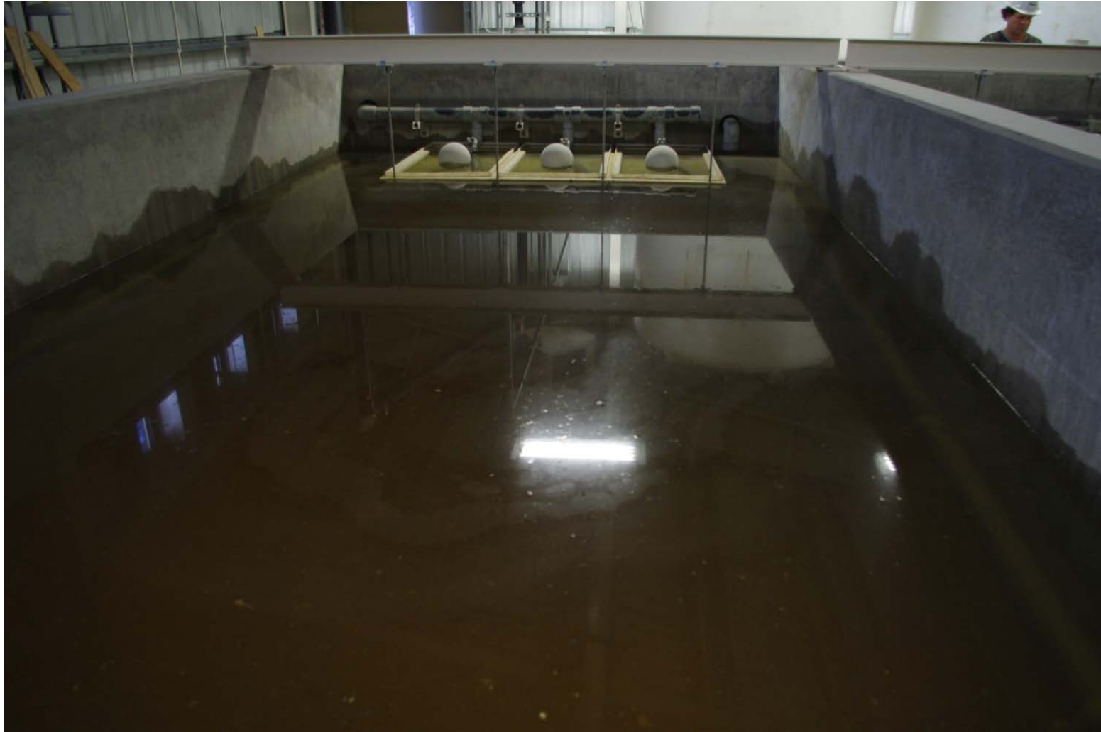
Operating filter in the Exshaw water treatment plant.
