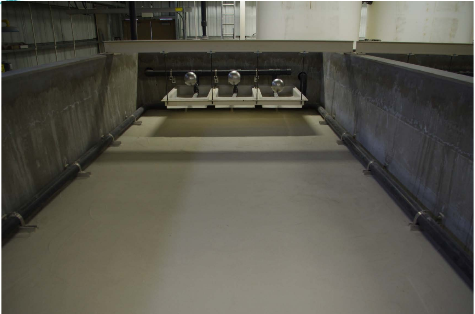
Interior of one filter cell in Exshaw water treatment plant.
