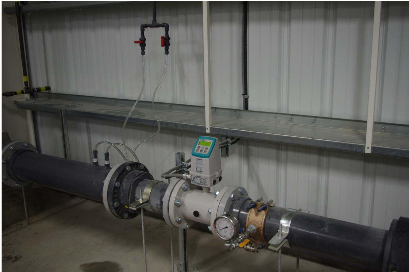
Flow metre and chlorine injection point for raw water entering Exshaw water treatment plant.
