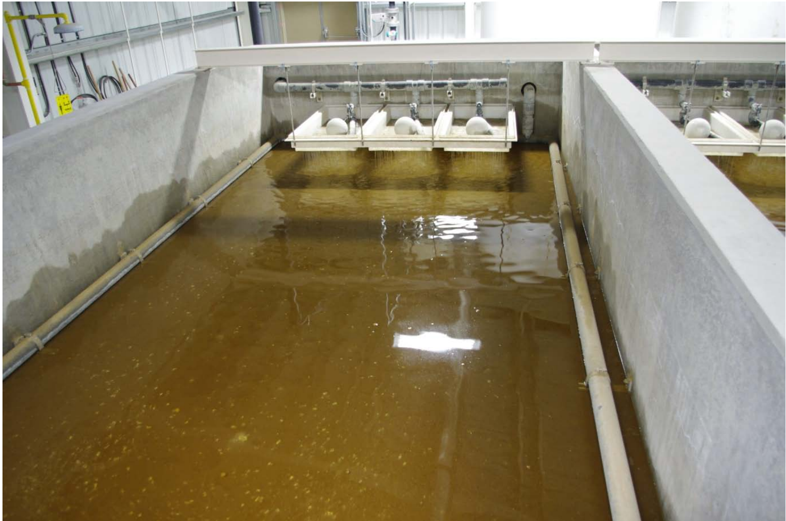
Filter after removal of backwash water.
