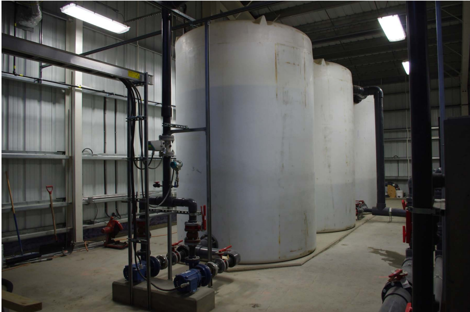
Three contact tanks and transfer pumps in Exshaw water treatment plant.
