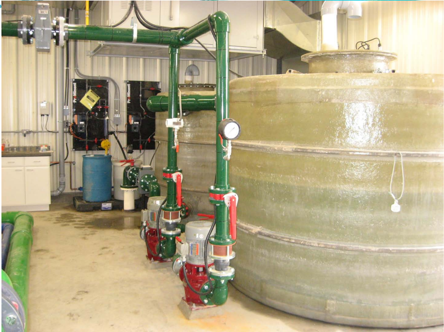
View of raw water inlet, contact tanks, transfer pumps and lab.
