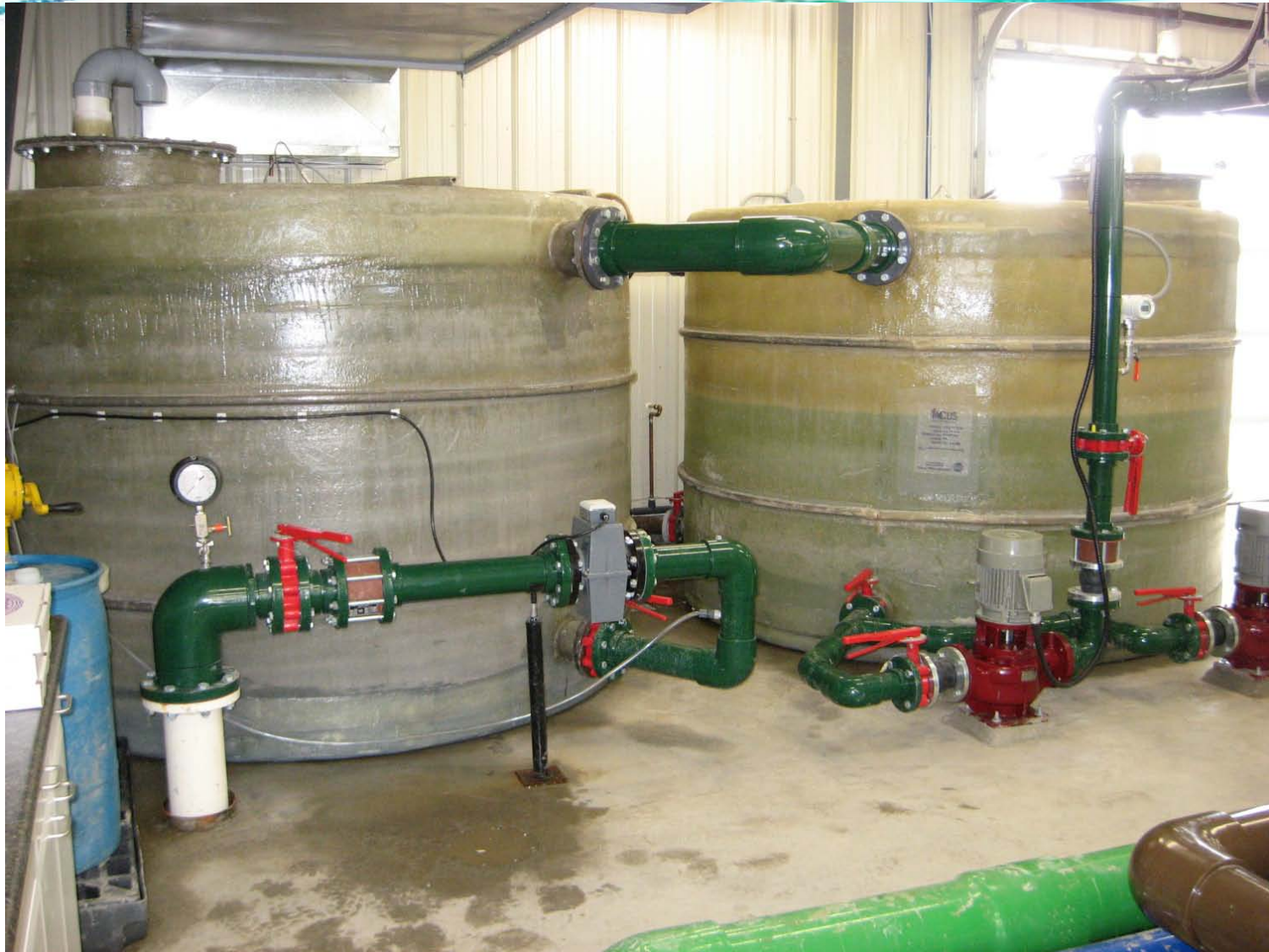
Two contact tanks – ensure formation of micro-flocs and transfer pumps.
