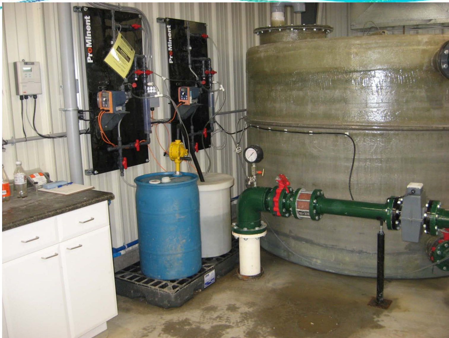
Inlet from well, flow meter and chlorine dosing equipment. (Note lab bench and equipment at left.)
