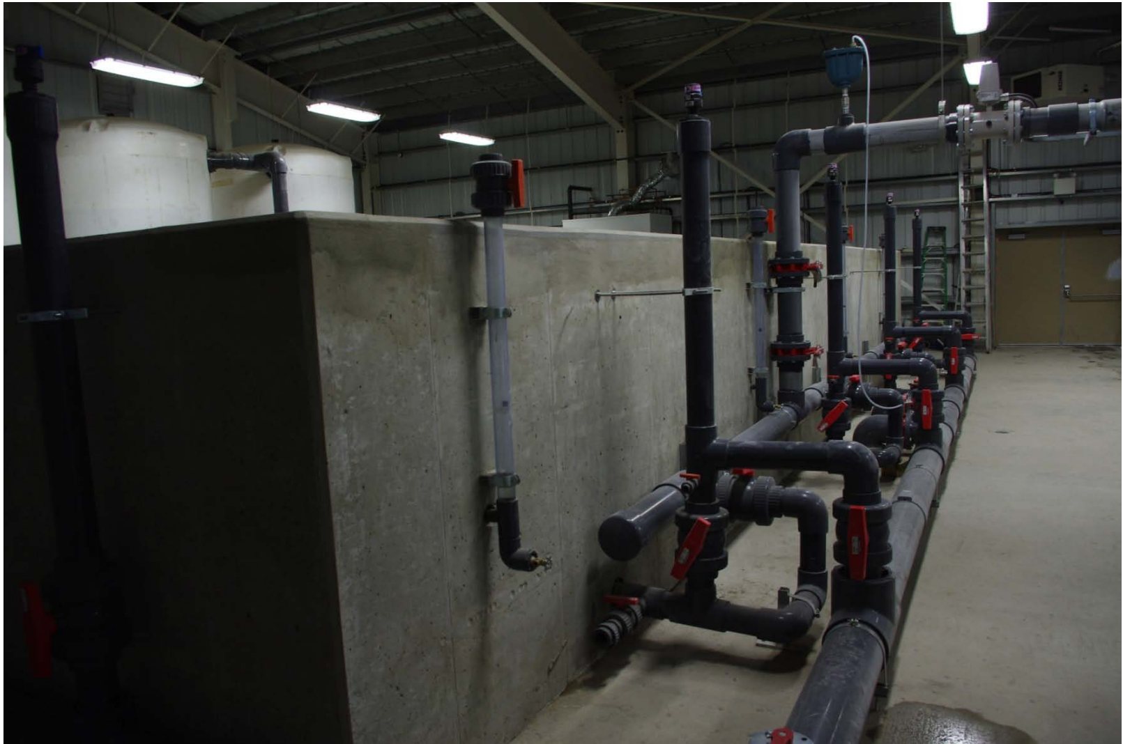
Filtered water outlet and backwash water inlet system.
