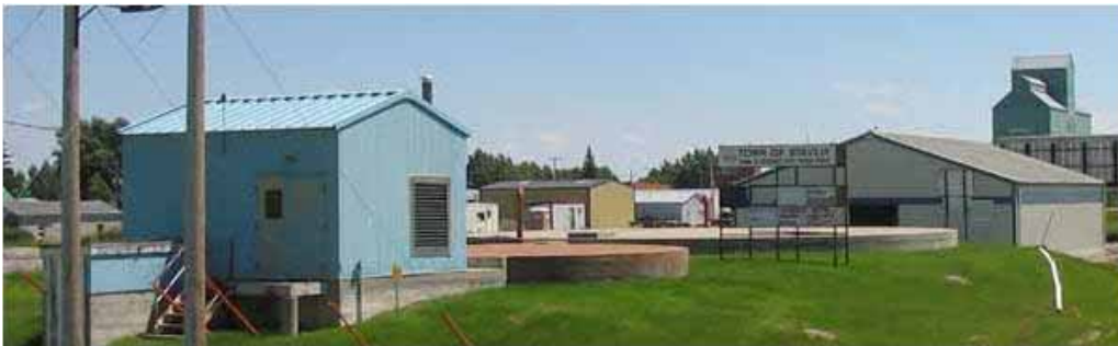
50,000 litres/hour MPSF based water treatment plant for manganese removal in Stavely, Alberta, Canada (pop 450) Above: exterior of plant and reservoir Below: cells prior to installation of media
