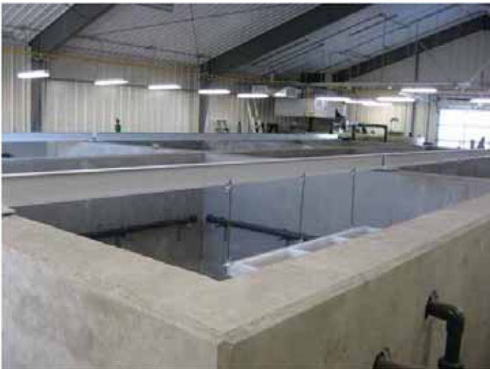
50,000 litres/hour MPSF based water treatment plant for manganese removal in Stavely, Alberta, Canada (pop 450) Above: exterior of plant and reservoir Below: cells prior to installation of media
